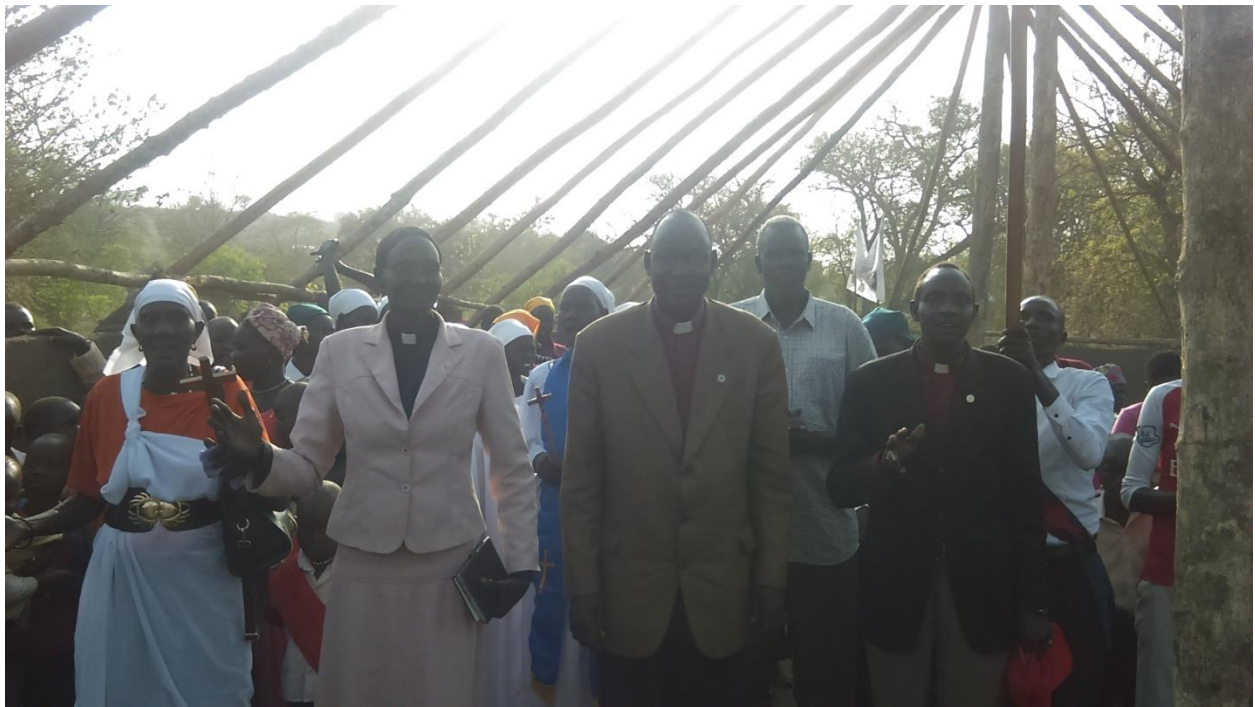
An unfinished Church building in Alere refugee camp: South Sudanese refugees' church officials have welcomed Bishop Elijah's missionary teams at Alere's settlements, saying they are happy to received Good News.
